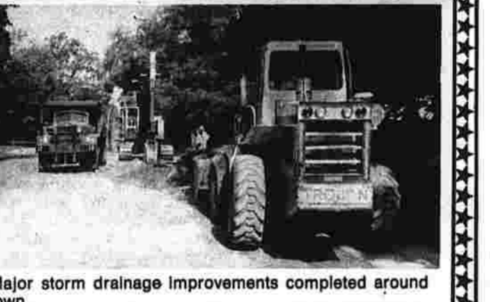
Major storm drainage improvements completed around town.
