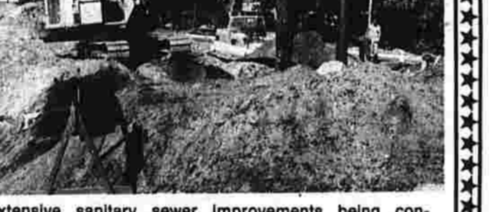
Extensive sanitary sewer improvements being constructed in North Manchester.
